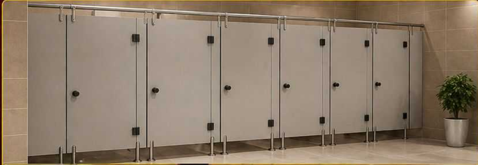
SAMPLE INSTALLATION – TOILET PARTITION CUBICLE
