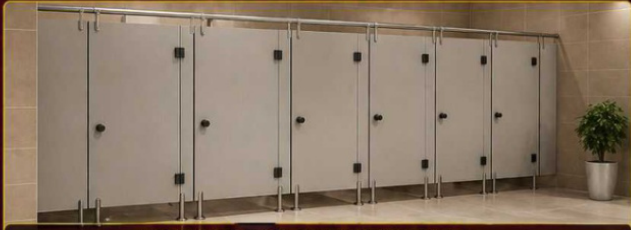
SAMPLE INSTALLATION - TOILET PARTITION CUBICLE
